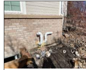
No protection on vents
